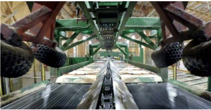
Red Stag's huge new CLT plant at Rotorua will be commissioned in early 2021.
