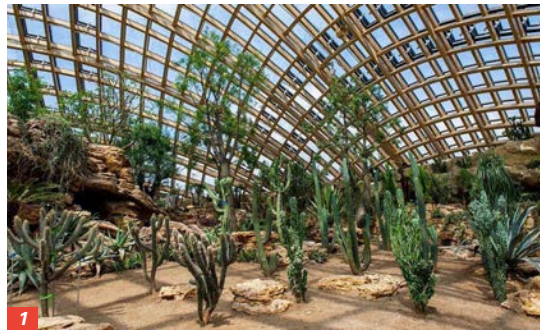
1/ China's garden domes... world's longest clear-span timber grid shell. 2/ World's largest planetarium under a wooden geodesic dome.
