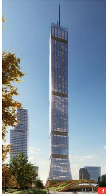
1/ The hybrid timber tower would be the tallest building in Canada at 105 storeys. 2/ Canadian concept... construction uses a patent-pending, prefabricated, composite hybrid timber floor system combined with a diagrid steel structure and concrete core that slashes embodied carbon.
