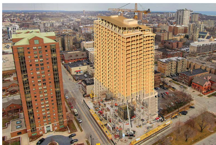
The 25-storey Ascent tower in downtown Milwaukee edges out Voll Arkitekter's Mjøstårne in Norway as the world's tallest mass-timber building.
