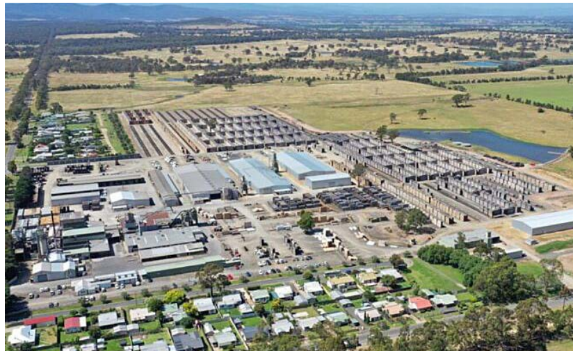
Funding will support the build of the specialised MASSLAM manufacturing facility.
