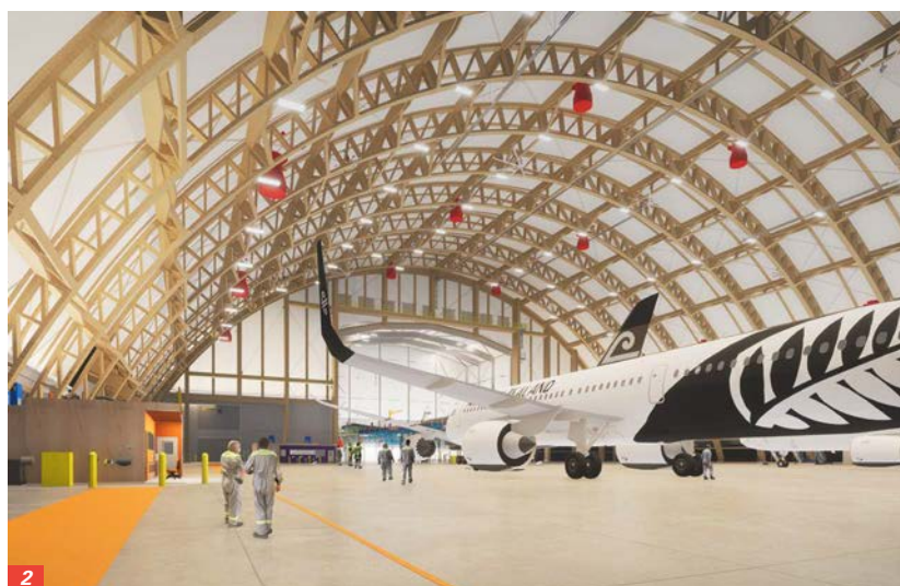
1/ Air New Zealand's Hangar 4: at 98 metres, it will be the largest single-span timber arch aircraft hangar in the southern hemisphere.
