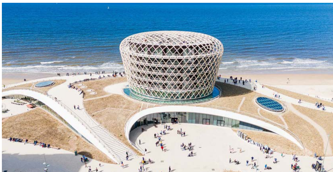
the new SILT coastal hotel and casino in Belgium with its stunning Accoya wood exterior. Image: courtesy Accsys
