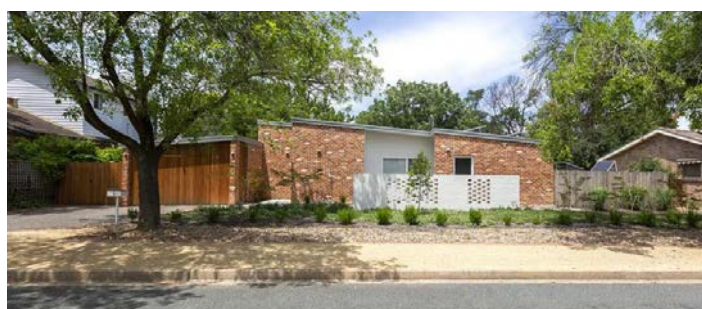
Oska's House was reimagined to create a more functional family home with the use of NatHERS energy modelling as well as repurposing salvaged materials. Image: HIA Australia
