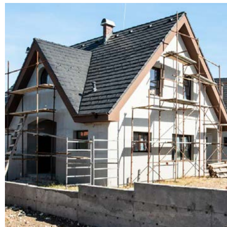
Strong economic conditions and lower cost of building is driving an increase in areas outside cap cities. Image: Shutterstock
