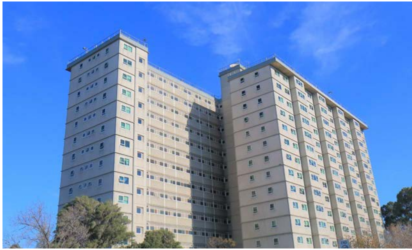
Social housing is important to help support low-income earners, domestic violence victims and those at risk of homelessness. Image: Shutterstock
