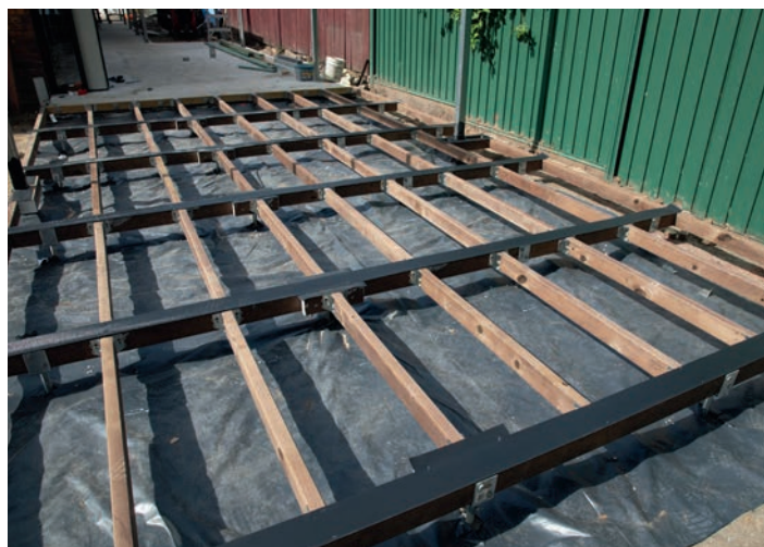
Being timber, TerraFrame is easy for installers to use on site. Adding joist tape can help to move water away from the top of the subframe.
