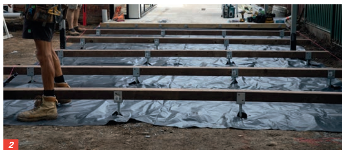
1/ TerraFrame from Woodhouse is a new H4 outdoor timber product suitable for a wide range of structural applications.
