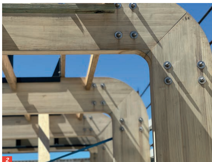
1/ 4-sided planer planing a beam. 2/ Curved Accoya portal frames in Sunshine Beach QLD.
