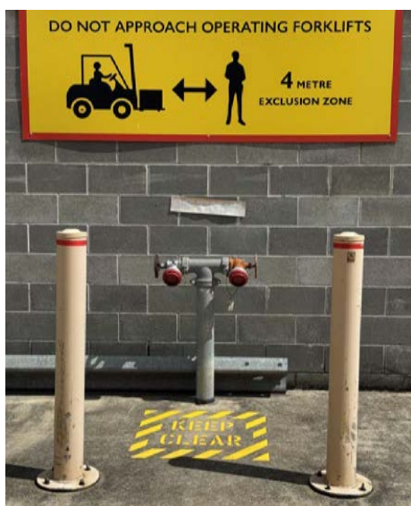
Bollards with signage are vital tools to assist the workplace with safety obligations. Image: Campbell McInnes
