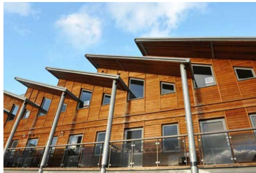
70% of new homes are detached. Gentle density is about allowing more land to be used for higher density dwellings such as townhouses and small scale apartments. Image: Shutterstock
